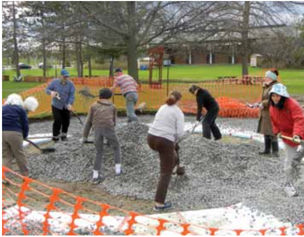
Garden members spread gravel over insulation panels. PHOTOS BY ED KUCERAK
