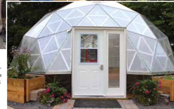
The Biodome Garden is the first of its kind in Ottawa. In addition to interior raised beds, the biodome structure has exterior raised beds for conventional crops
